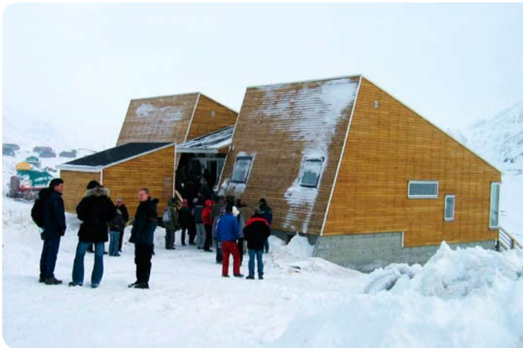
The inauguration of the Low Energy House in Sisimiut in April 2005
