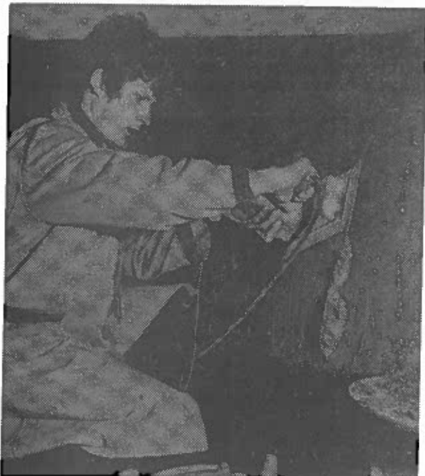
Fig.11 Building-up of ferro-cement
