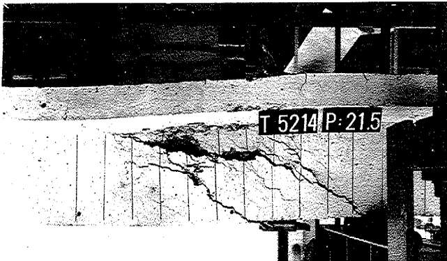
Figure 5.2.2: Failure of Beam No. T5214
