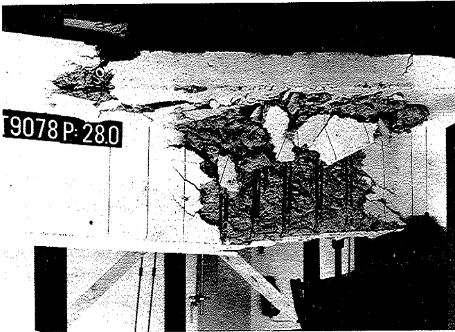
Figure 5.1.2: Second failure of Beam No.T9078
