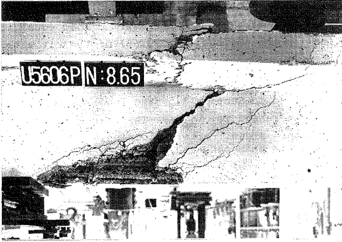
Fig.6.2: Fatigue failure of stirrups. V_{\max} = 0.5 V_u
