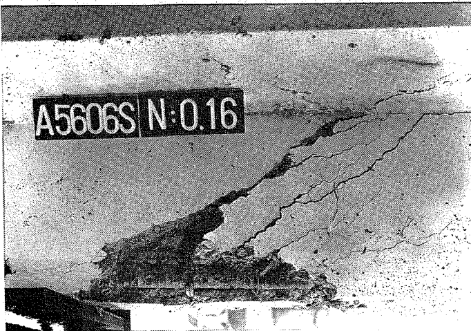
Fig.6.5: Fatigue failure of stirrups. V_{\max} = 0.62 V_u
